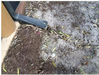
One downspout extension is crushed but the gutters are in good condition otherwise.
