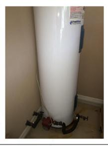
The water heater is working but does have a small leak. The water heater will need to be replaced to fix this problem.
